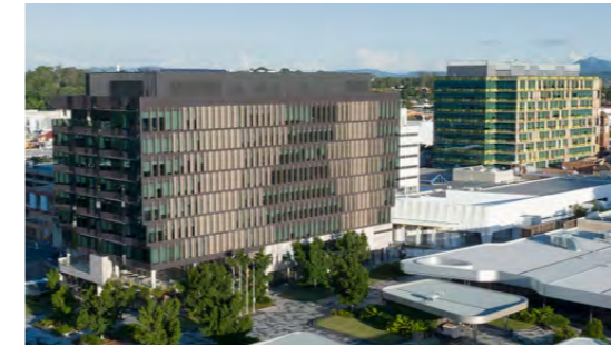
IPSWICH CBD DEVELOPMENT: $250M Ipswich CBD redevelopment will act as the catalyst for Ipswich City to cement itself as one of the most exciting urban and economic growth zones in Australia.
