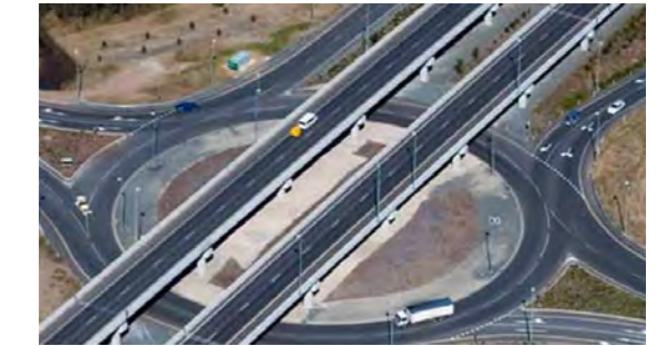
IPSWICH MOTORWAY UPGRADE: $400M upgrade project over a 7km section of motorway between Darra and Rocklea to improve traffic flow to Ipswich.
