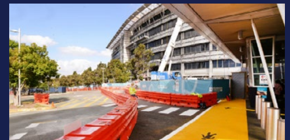
Princess Alexandra Hospital Cladding
